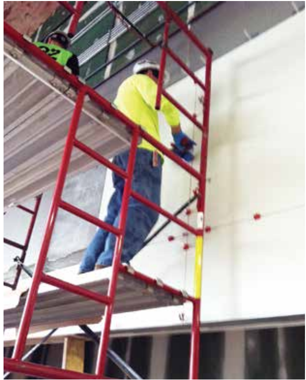
Prepared panels installed using Tuscan Leveling System.
