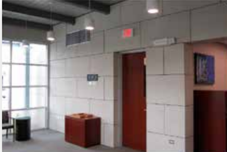
Ventilated rainscreen mockups in IMI's Addison training center helped lead to the use of this system on the interior and exterior walls on the First Bank and Trust in Skokie, Illinois, installed by Trowel of Excellence™ certified contractor DTI of Illinois.
