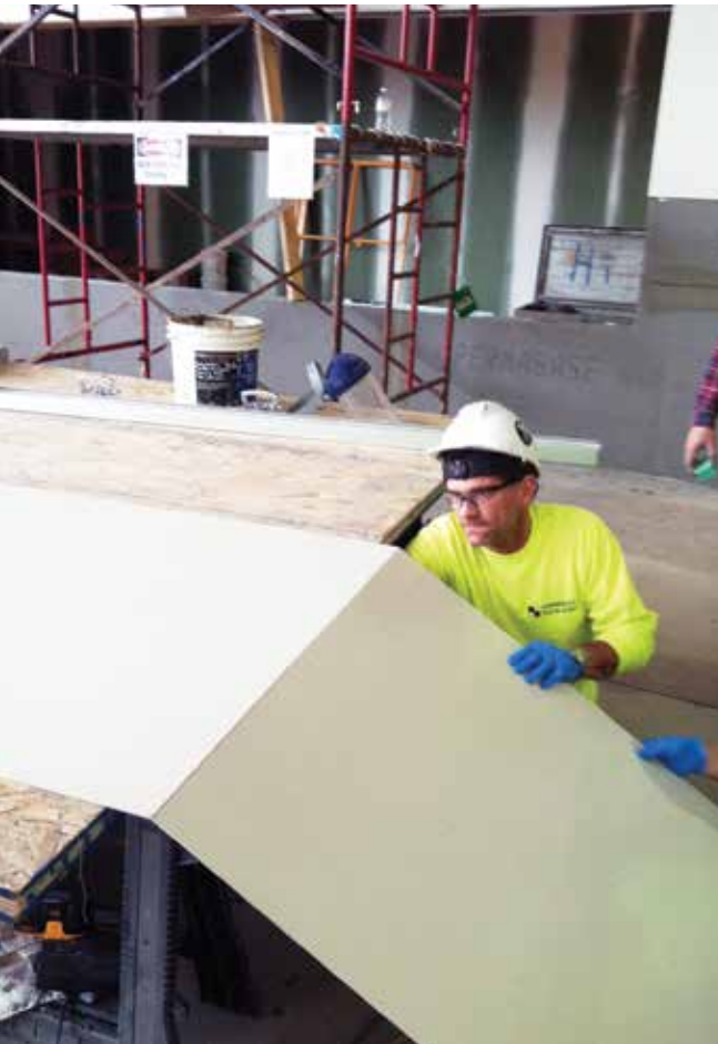
Once cut, the thin porcelain panel cleanly snaps in half.
