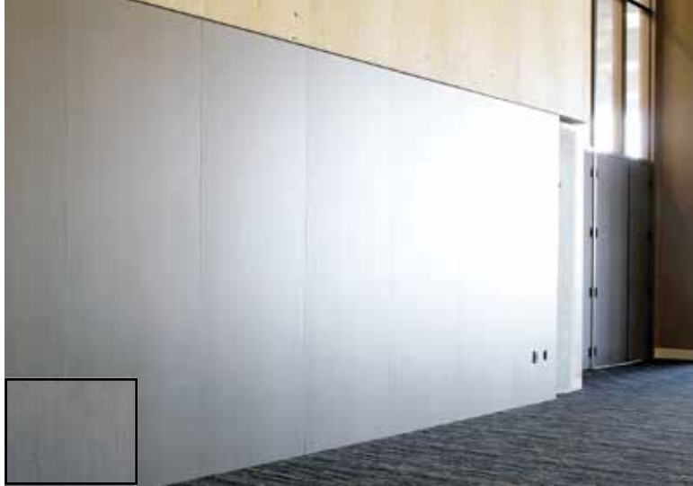
Installed 10' x 3' Laminam panels. Insert shows textured panel face.
