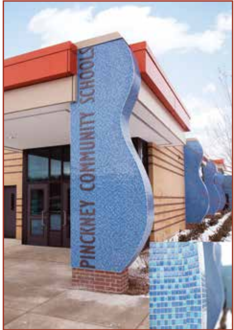
Curved pillars featuring glass tile and designed to resemble a cello presented unique installation challenges.
